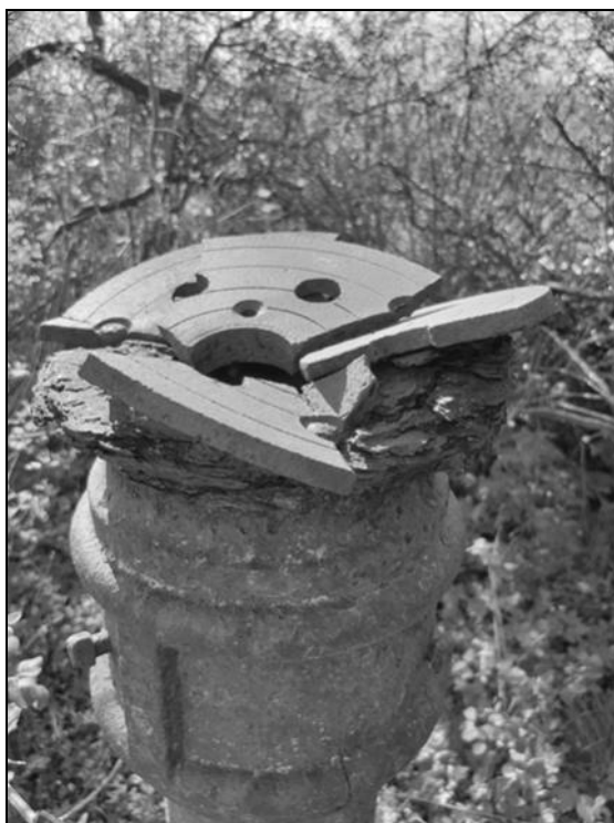
Fig. 3: Remains of the telescope pillar and mount; the walls and roof are completely removed and only sections of the poured concrete floor are left. (Authors)
